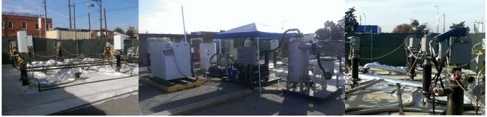
In Situ Thermal Remediation was used to successfully treat benzene, TPH-d, TPH-mo, BaP, and Naphthalene from a former gas plant in EPA Region 9. Gas Thermal Remediation (GTR™), using Thermal Conductive Heating (TCH), raised the temperature of the soils in the treatment zone of the former MGP site to an average temperature of approximately 325 degrees Celsius.
